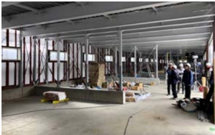
Building safety assessment
